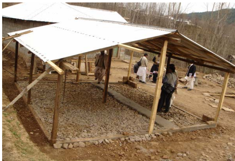
After the completion of structure & roof shelter is ready for the construction of sidewall
