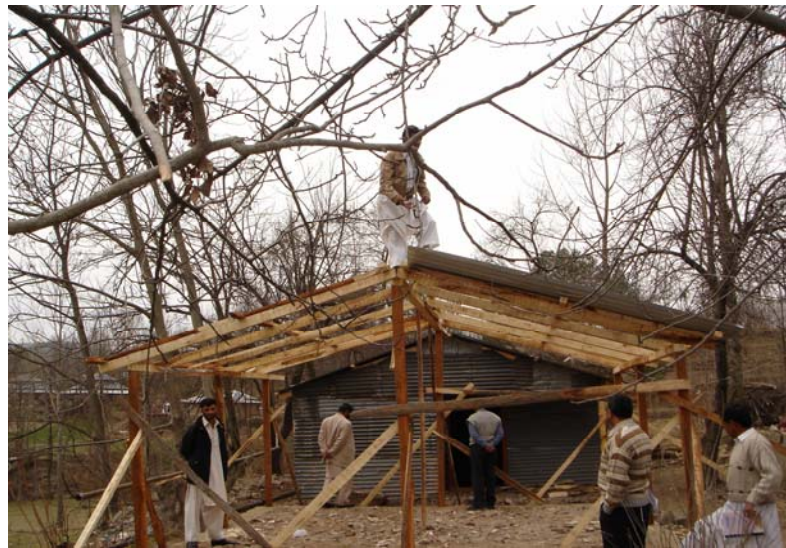
After the completion of structure CGI sheets are being used for Roofs
